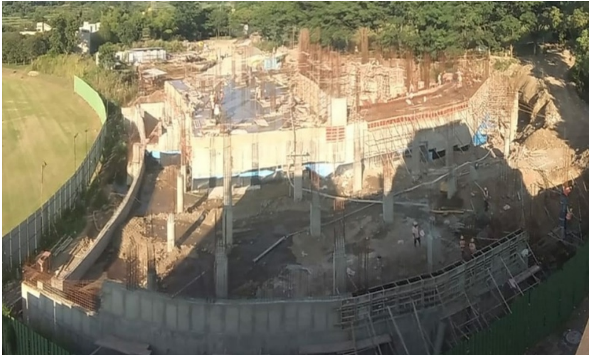
Figure 22: A new auditorium- under construction in 2021
